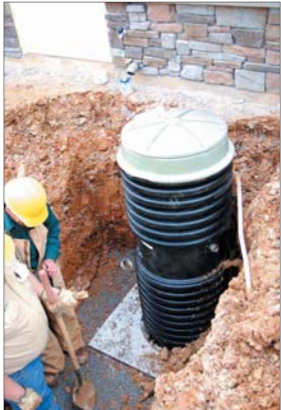
*Individual grinder pumps installed at each site push slurry of wastewater from homes and other sites to the central sewer or treatment plant.*
