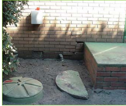
Figure 4. Installation of pump unit & switchboard completed.
