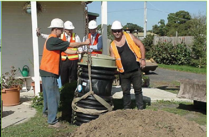
Figure 3. Lowering the unit into position
