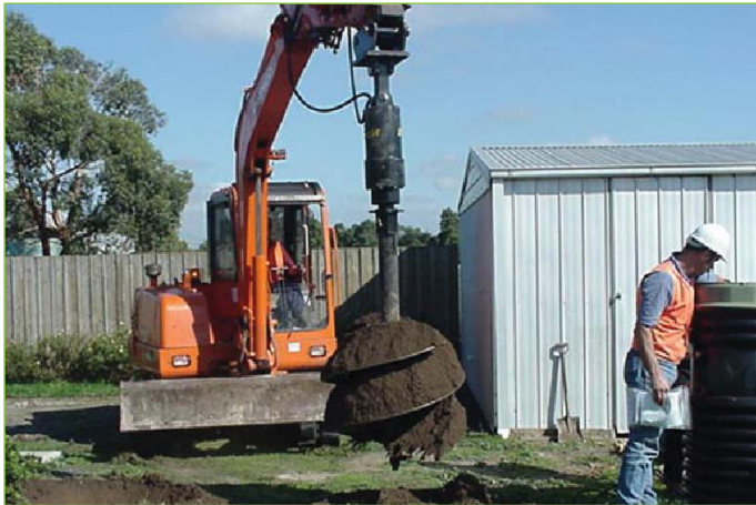
Figure 2. Installation by auger
