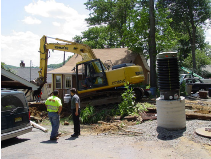
Figure 5 – Grinder Pump Installation
