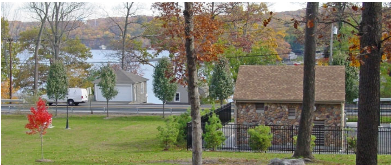
Figure 3 – Lakeside Pump Station-Modic Park
