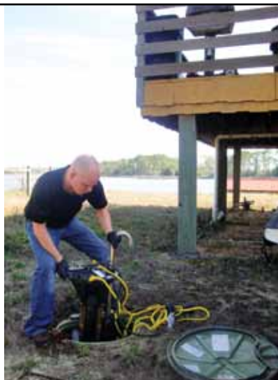
Carrabelle's pressure sewer system uses small-diameter pipes and grinder pumps installed at each home.
