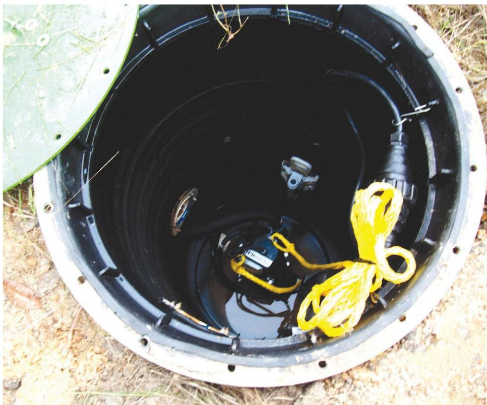
Top view of E/One grinder pump station.
