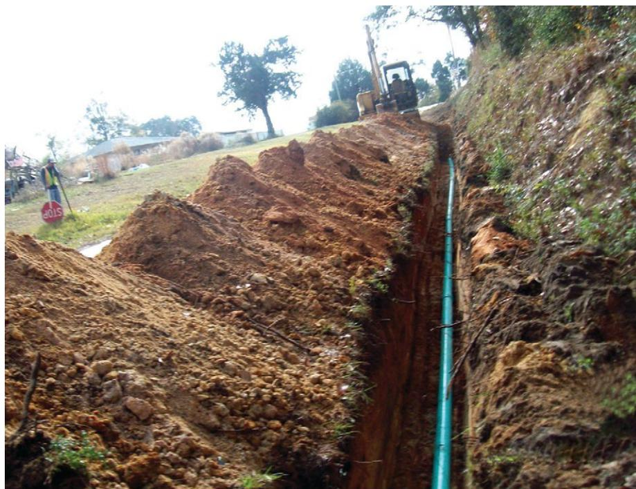
Pressure sewers use small-diameter pipelines, minimizing environmental disruption.
