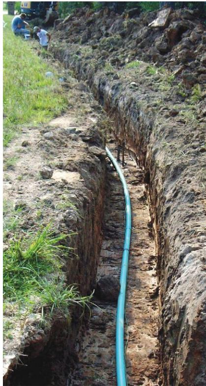
*Small pressure sewer mains require only small trenches during installation.*
